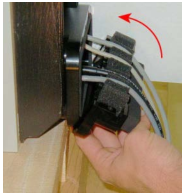
Figure 9-5. Installing Lower Flange
